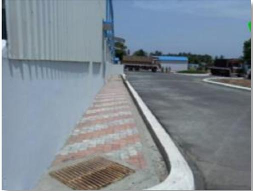
*Fig.6.3.7.Premises tarred and concreted to avoid dust*
