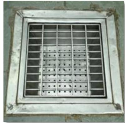
Fig.6.3.23.Covered drains to prevent insects and rodents
