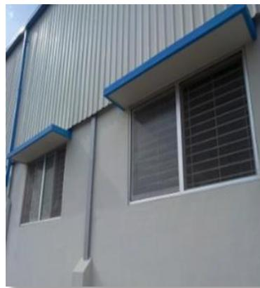
Fig.6.3.25.Nets and mesh on windows to avoid pest entry
