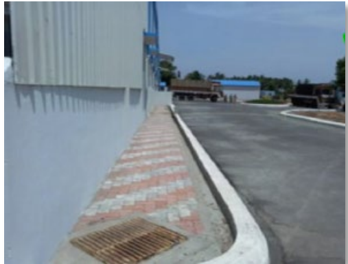
Fig.6.3.7.Premises tarred and concreted to avoid dust
