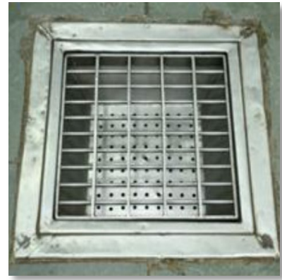
Fig.6.3.23.Covered drains to prevent insects and rodents
