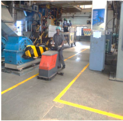
Fig.6.3.21.Special stone flooring to avoid slipping and easy to clean
