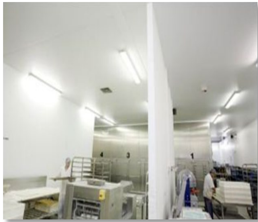
Fig.5.3.28. Proper lighting facility in the work area
