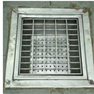
Fig.6.3.23. Covered drains to prevent insects and rodents
