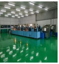
Fig.7.3.22.Epoxy and smooth flooring, easy to clean and avoids dust accumulation and microbial contamination
