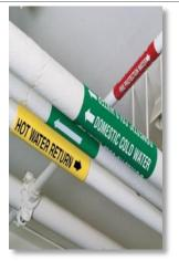
Fig.7.3.34.Color coding of water pipes to avoid contamination
