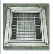
Fig.7.3.23.Covered drains to prevent insects and rodents
