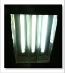
Fig.7.3.26.Covered lights in the production area
