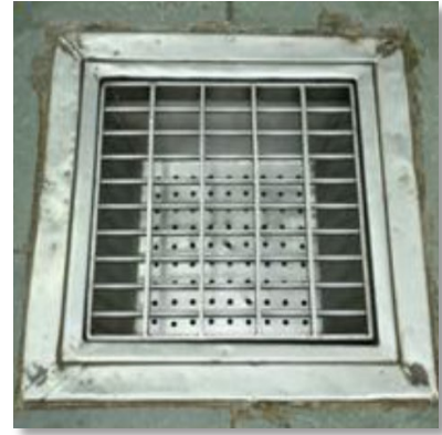
Fig.5.3.23. Covered drains to prevent insects and rodents
