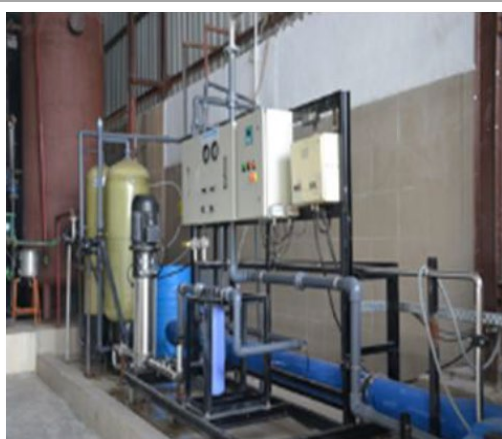
Fig 5.3.4. Waste water disposal system/effluent treatment plants
