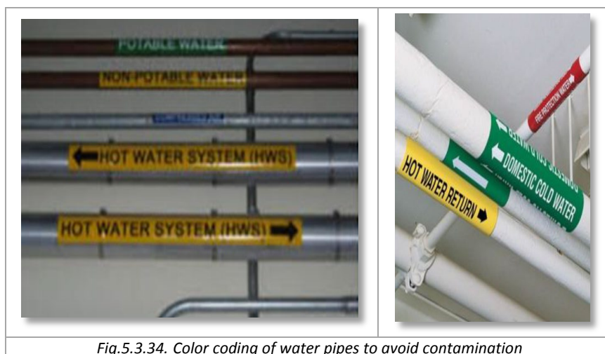
Fig.5.3.34. Color coding of water pipes to avoid contamination
