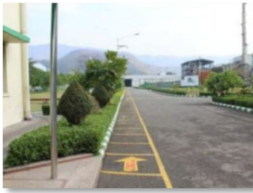
Fig.6.3.13. Clearly defined walkway water stagnation near the surroundings
