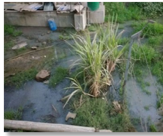
Fig.6.3.14. Avoid vegetation growth near the premises
