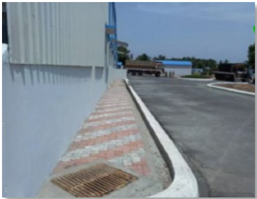
Fig.6.3.7. Premises tarred and concreted to avoid dust
