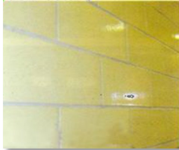
Fig.6.3.16. Walls: clean, durable, impervious to moisture
