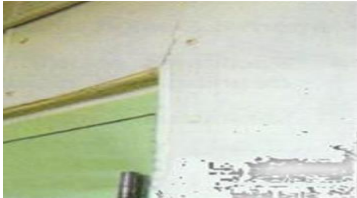
Fig.7.3.17.Avoid Cracks on walls as it allow bacteria and moulds to accumulate
