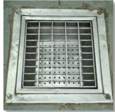
Fig.7.3.23.Covered drains to prevent insects and rodents
