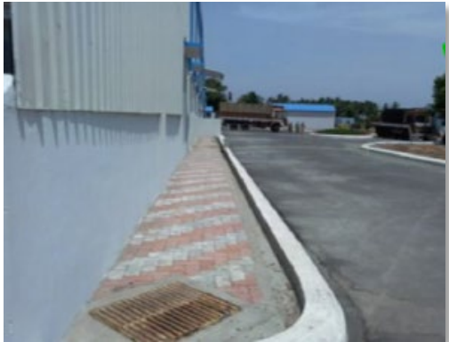
Fig.6.3.7.Premises tarred and concreted to avoid dust
