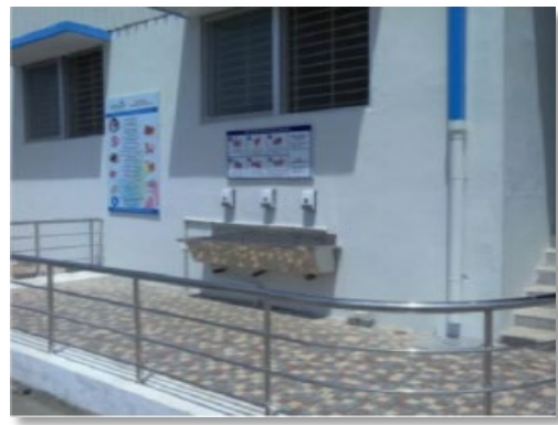
Fig.6.3.8.Entrance with hygiene station
