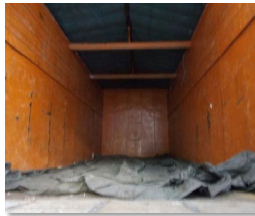
Fig.6.3.29. Vehicle inspection before loading
