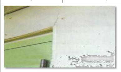
Fig. 6.3.17.Avoid Cracks on walls as it allow bacteria and moulds to accumulate
