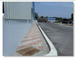
Fig.6.3.7.Premises tarred and concreted to avoid dust
