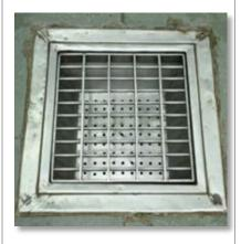
Fig.6.3.23.Covered drains to prevent insects and rodents
