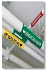
Fig.6.3.34.Color coding of water pipes to avoid contamination
