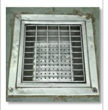
Fig.6.3.23.Covered drains to prevent insects and rodents
