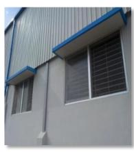
Fig.6.3.25.Nets and mesh on windows to avoid pest entry
