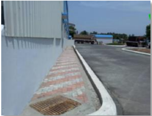
Fig.6.3.7.Premises tarred and concreted to avoid dust
