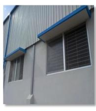
Fig.7.3.25.Nets and mesh on windows to avoid pest entry
