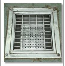
Fig.7.3.23.Covered drains to prevent insects and rodents
