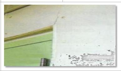
Fig.7.3.17.Avoid Cracks on walls as it allow bacteria and moulds to accumulate
