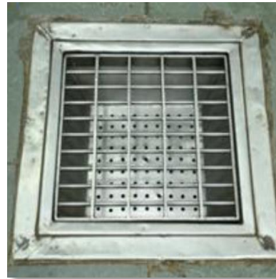
Fig.6.3.23.Covered drains to prevent insects and rodents
