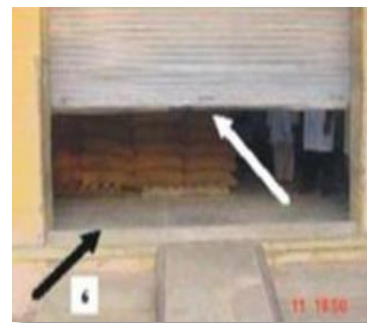
Gap in between shutter and floor
