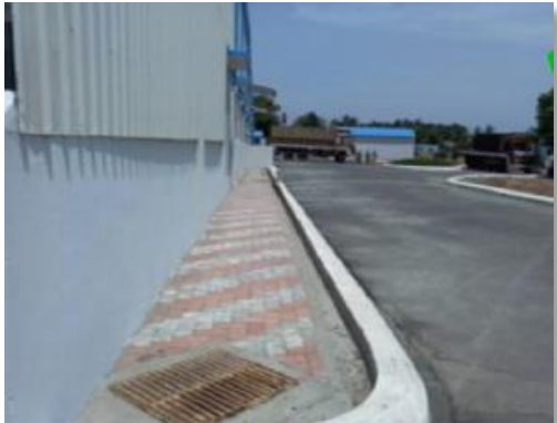
Fig.6.3.7.Premises tarred and concreted to avoid dust
