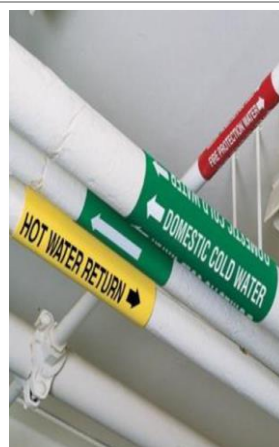
Fig.6.3.34. Color coding of water pipes to avoid contamination
