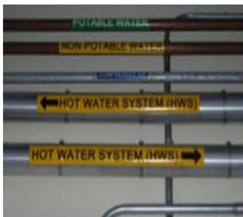
Fig.6.3.34. Color coding of water pipes to avoid contamination
