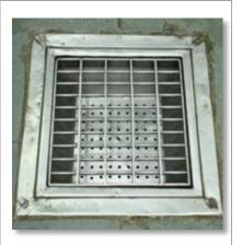
Fig.5.3.23. Covered drains to prevent insects and rodents
