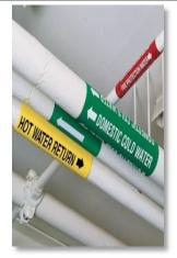
Fig.5.3.34. Color coding of water pipes to avoid contamination
