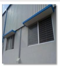
Fig.5.3.25. Nets and mesh on windows to avoid pest entry
