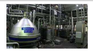
**Pasteurization:** Milk will be subjected to the pasteurization in a continuous flow. The milk enters in the pasteurizer at 4 deg C and leaves at 4 deg C. Milk pasteurizer is available with 90 - 95 % regeneration efficiency.
